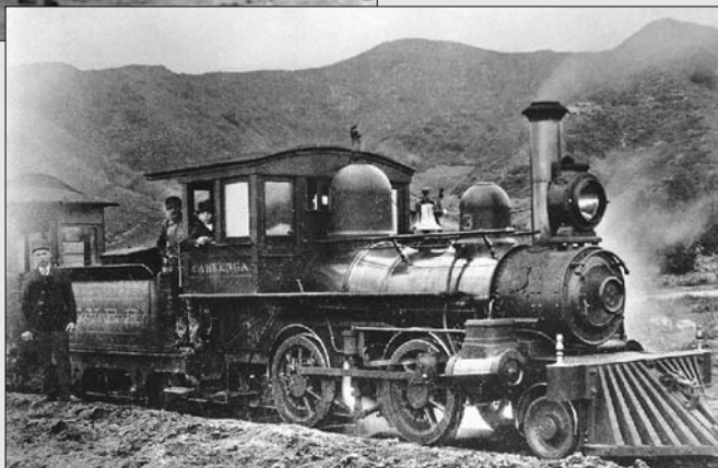
Right: The little engine is standing on Sunset Boulevard at Laurel Canyon in the year 1893. The railway was responsible for the unusual configuration of Crescent Heights which was used as a connection to the Santa Monica Boulevard steam dummy line. There was a rock quarry just west of Laurel Canyon. Trains hauling rocks required large radius curves to turn onto Crescent Heights at Sunset and again at Santa Monica Boulevard. Those curves are still visible to this day.
